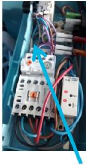
Non-modular units: disconnect red output cable to compressor contactor.
