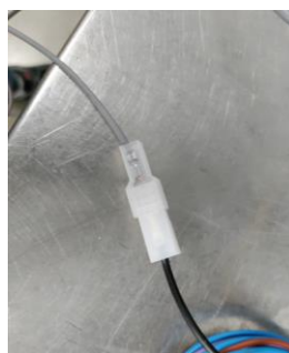
Connection Gray Cable #12 and Black Cable #1
